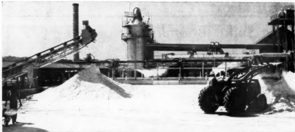
MAKING SULFUR. —This plant of Petroleos Mexicanos processes Poza Rica field gas, turns out 137 tons per day.
